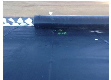
CQA processes give assurance via damage control systems
